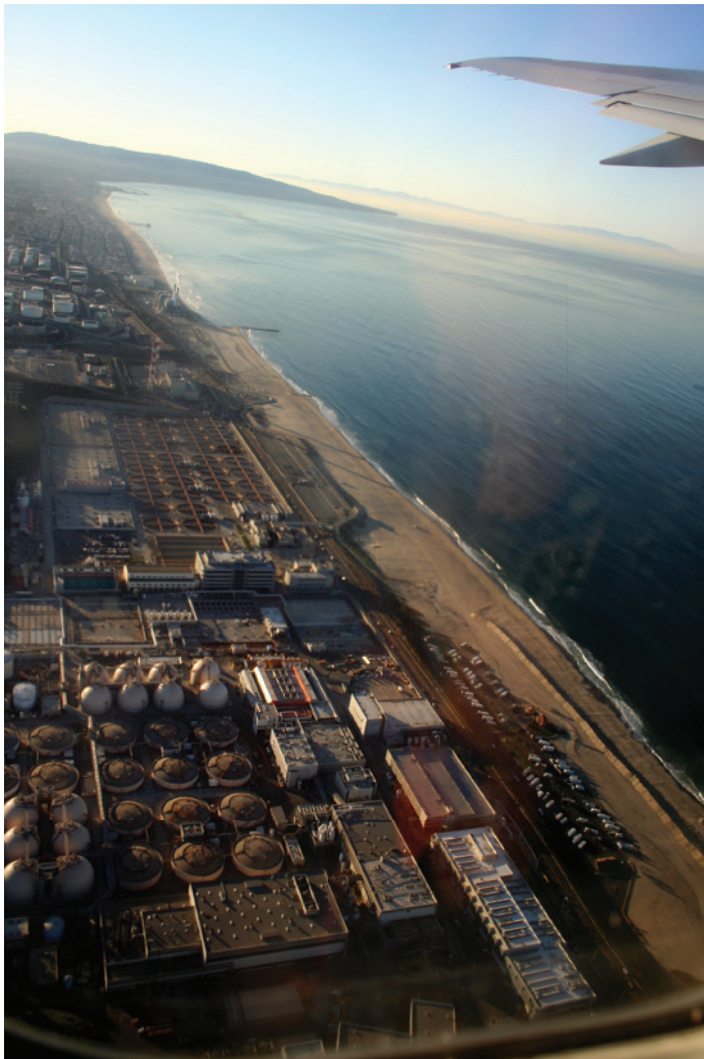
FIGURE 16B2-1 Sewage treatment plants are often located on the water's edge. This large secondary-treatment, the Hyperion plant in Los Angeles is located on a prime stretch of Pacific Ocean beach just west of Los Angeles International Airport.
